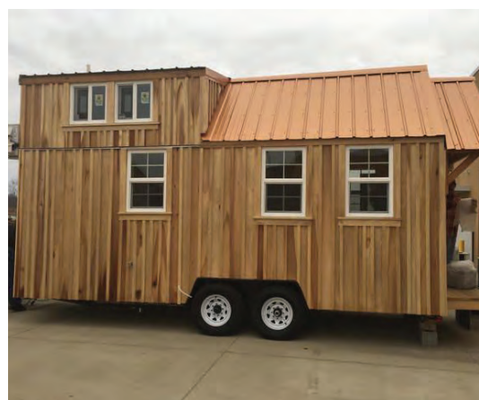
A Tiny Home constructed by Simulated Workplace student employees from Mingo Central High School
