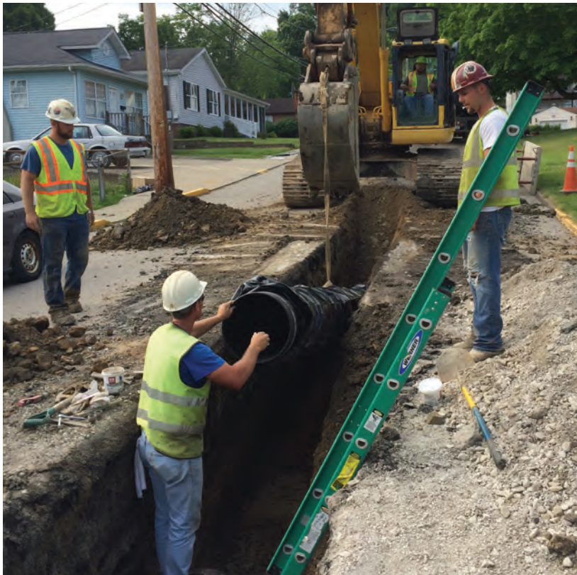
A crew installs a 16-inch water line along Henson Street in South Charleston. The new line is part of a $1.1 million water infrastructure upgrade project by West Virginia American Water
