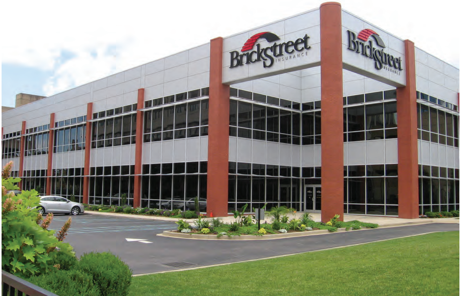
BrickStreet Insurance began its historic role as West Virginia's first private workers' compensation carrier in 2006
