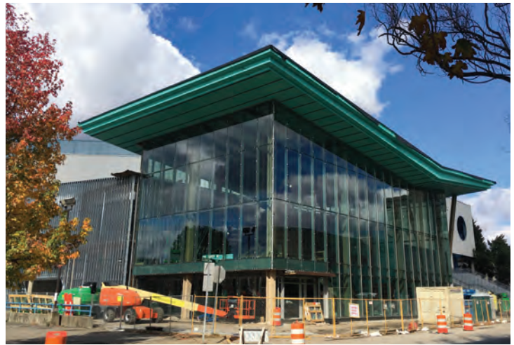
Renovation on the Charleston Civic Center
