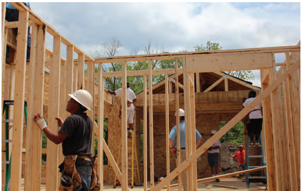
The Dan Ryan Builders and Habitat for Humanity Blitz Build
