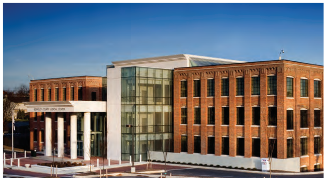
Berkeley County Judicial Center, Martinsburg, West Virginia
