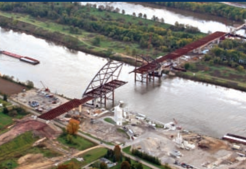
Early construction of the $120 million, tied-arch Blennerhassett Island Bridge, which is expected to open to traffic this summer.
