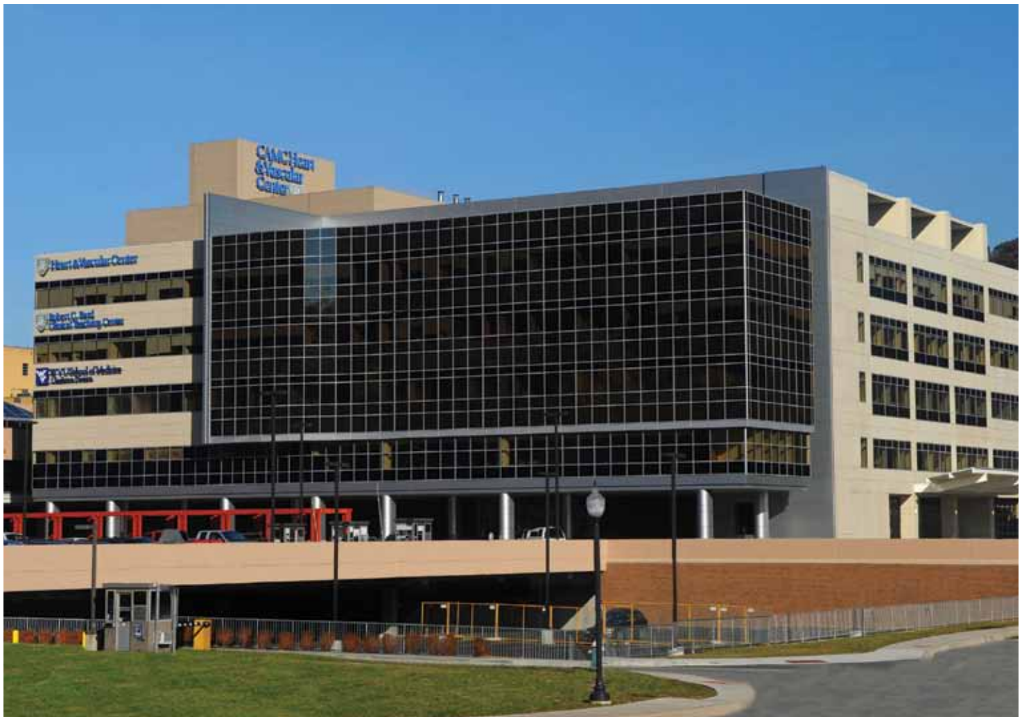
The new CAMC Heart and Vascular Center in Charleston, West Virginia
