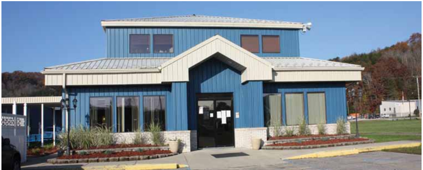
The Lincoln County WELL (Wellness, Education, Lifestyle and Learning) Center, built in 2004
