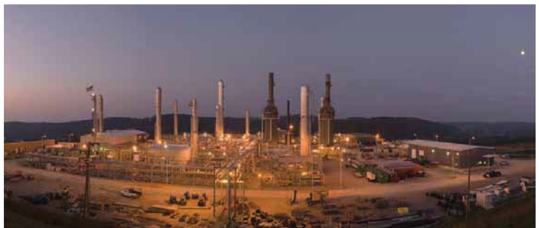
The Liberty Segment at the Houston Processing Facility in Houston, Pennsylvania
