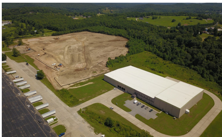
Rough grubbing and grading of a site in Parkersburg to make it more appealing to future site selectors.
