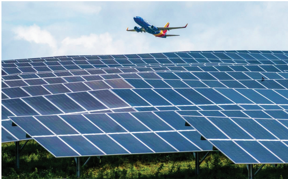
Taking flight over IMG's solar system on the southside of the Pittsburgh International Airport. The array is owned and operated by IMG and provides power to 23 separately metered airport facilities.
