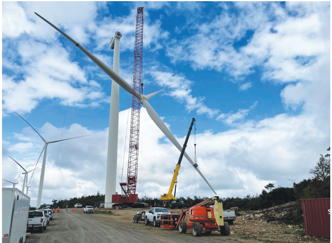
Upgrades to the Pinnacle Wind Farm near Keyser in West Virginia's Mineral County.
