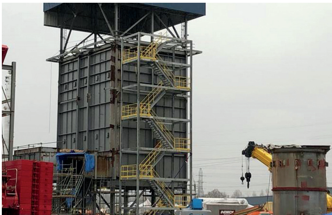
New stair tower for H-11-1 Reformer in Unit 1000 at Liberty One site
