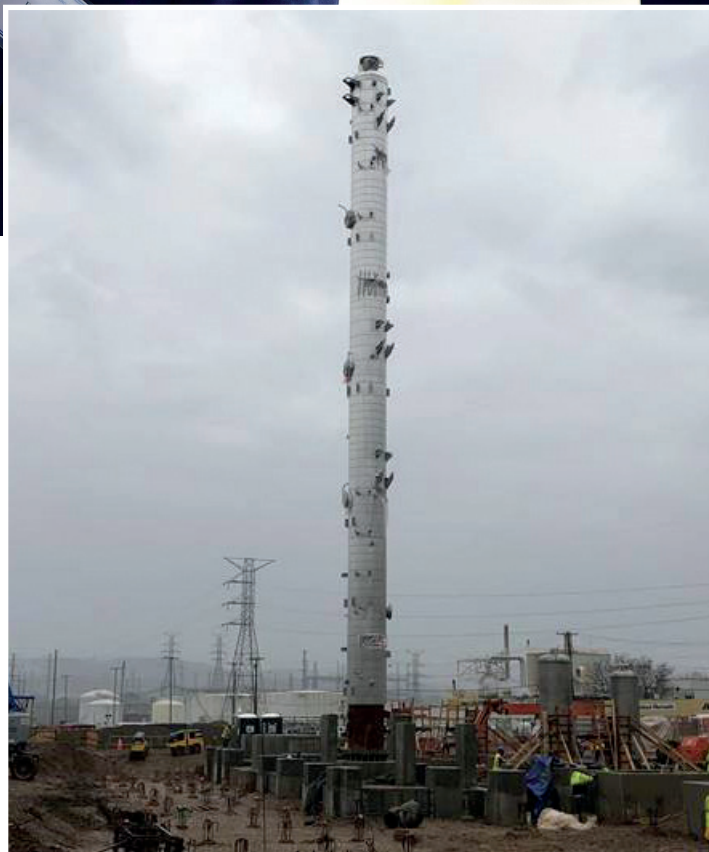
Distillation Tower T-3301 installed on foundation in Unit 3000 at Liberty One site
