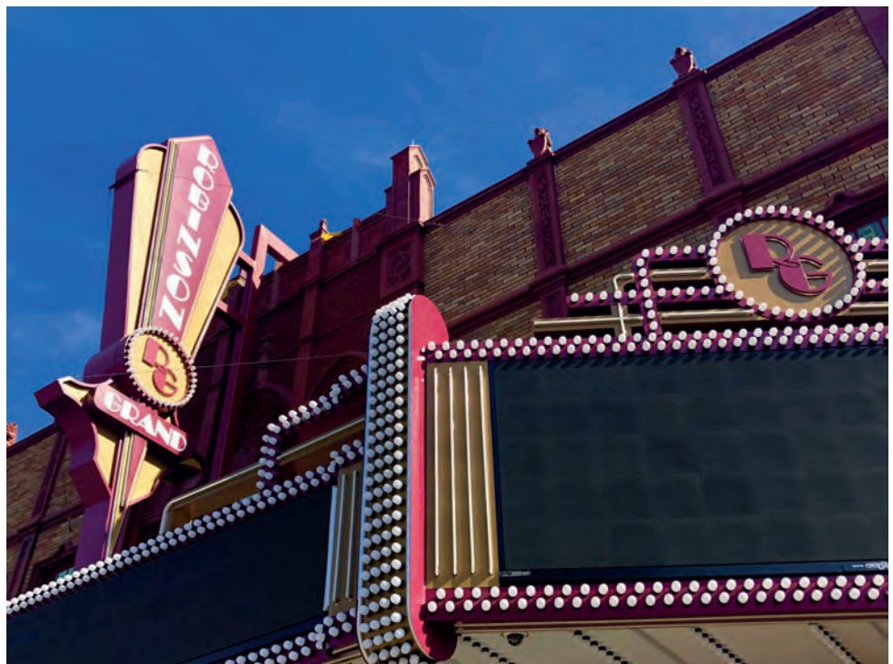
The Robinson Grand Theater in Clarksburg, West Virginia first opened its doors on February 7, 1913. After decades of vacancy, the restoration and renovation of the Robinson Grand was completed in the spring of 2018.
