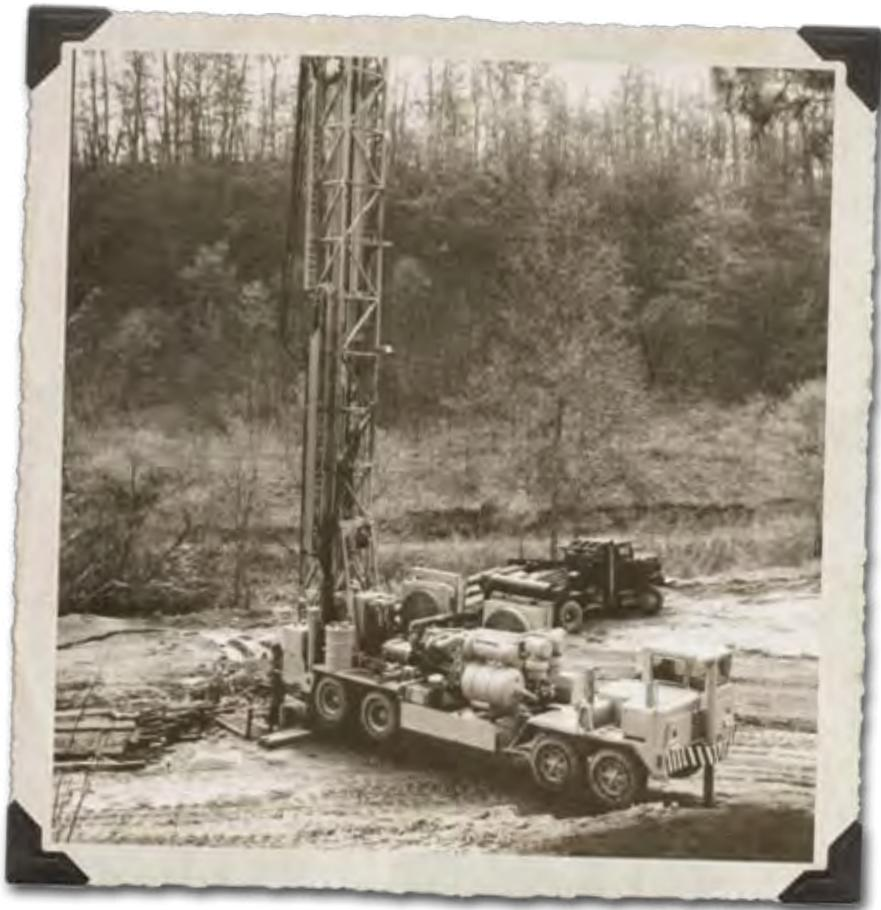
*The J. W. Kinzer Drilling Company took this Ingersoll-Rand RD-20, 110,000 lb. pullback rig to a new depth – 7,020 feet – in just seven days. The company achieved success by using hammer bits and aluminum drill pipe.*
