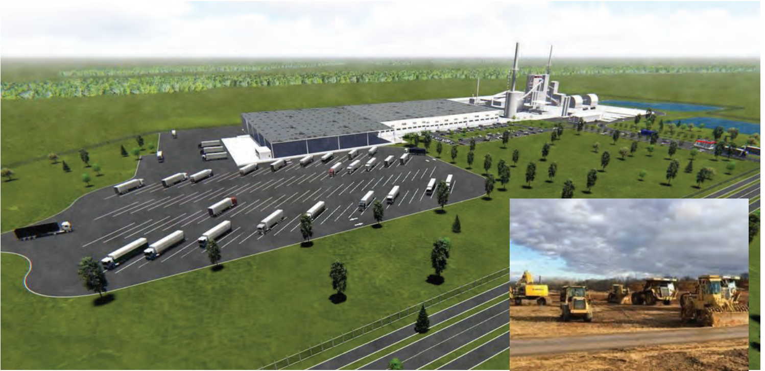
Above: Artist rendering of the Rockwool manufacturing facility in Ranson, West Virginia, scheduled for completion in 2020. Inset: Rockwool site preparation
