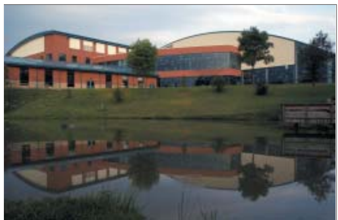
WVU's $34 million Student Recreation Center
