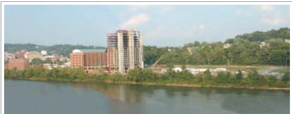
Among the many improvements taking place in North Central West Virginia is the development on Morgantown's Wharf District along the Monongalia River. The $186 million waterfront project includes the Caperton Trail, the 18-floor Radisson Waterfront Hotel and Conference Center, the Hazel Ruby McQuain Park and the WVU Visitors Resource Center.
